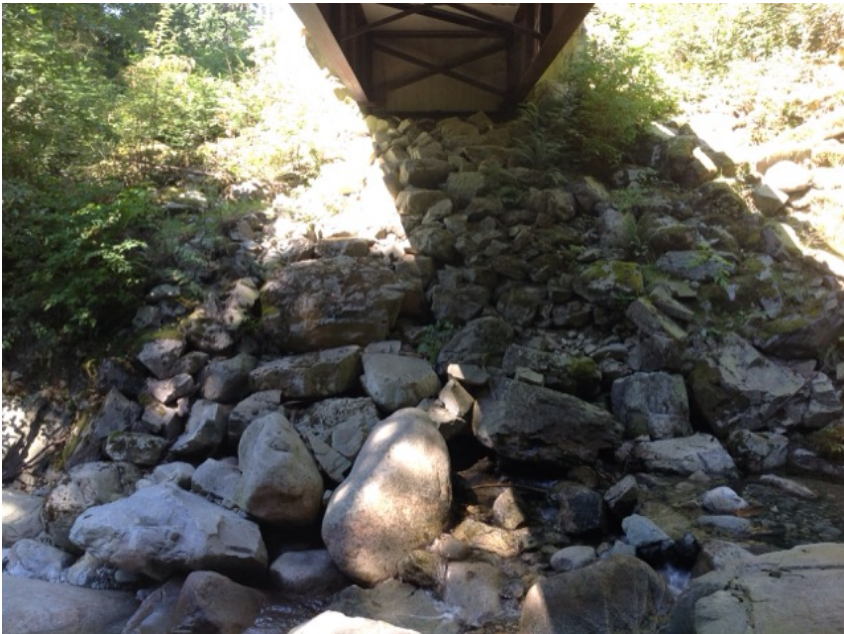
Right Bank Abutment when facing downstream
