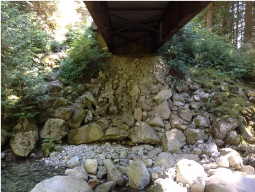
Left Bank Abutment when facing downstream
